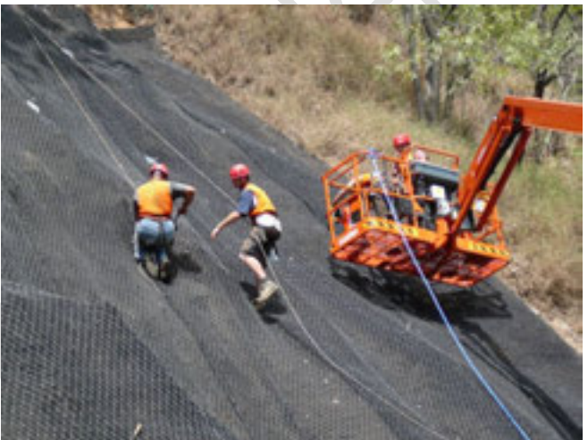
Above: Main Roads(Road Tek) - Rock Fall netting, diversion drains erosion controls & other land stability rectification systems installation on a slip at Buchans Point
