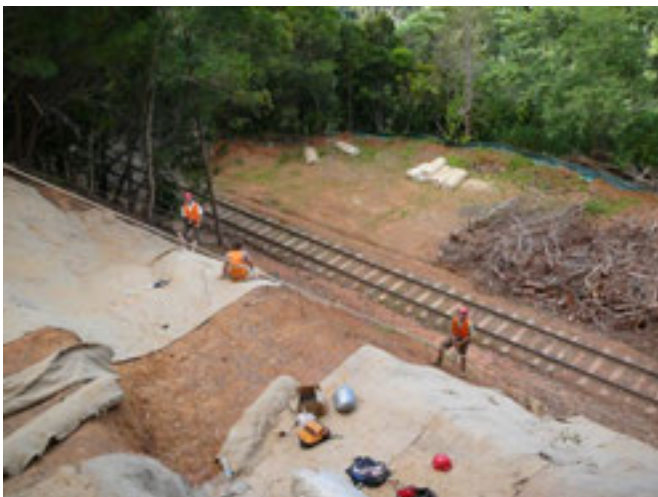
QR - Jute matting installation for on a slip near Barron Falls
