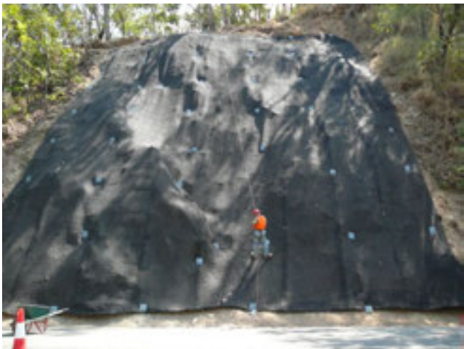
Above: Main Roads(Road Tek) - Rock Fall netting, diversion drains erosion controls & other land stability rectification systems installation on a slip at Buchans Point
