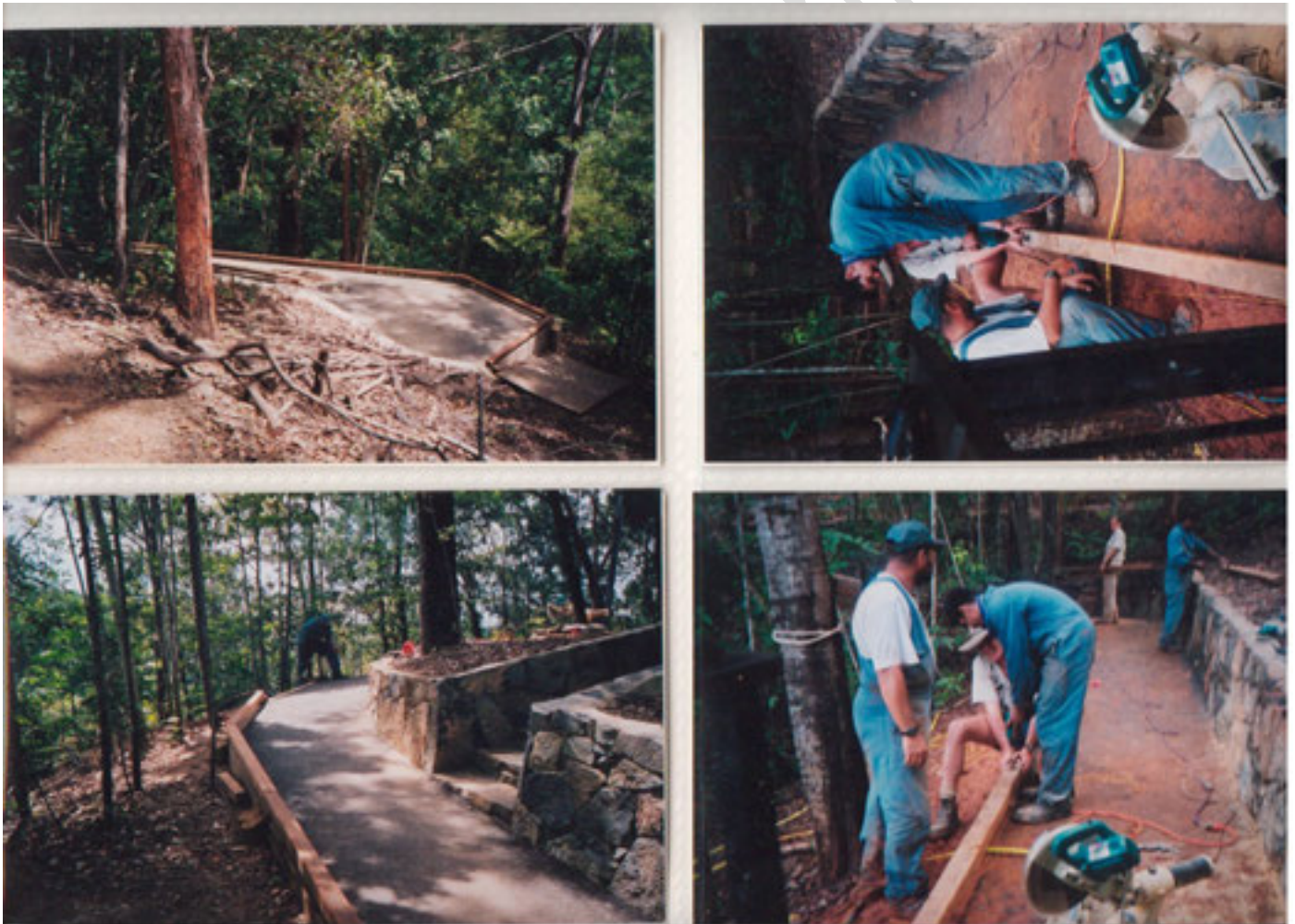
Construction of the boardwalk & on ground pathway at Barron Falls
