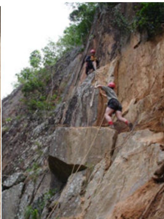
Cairns Regional Council: Dangerous rock removal (scaling) above Macka's Bluff in Lower Barron Gorge
