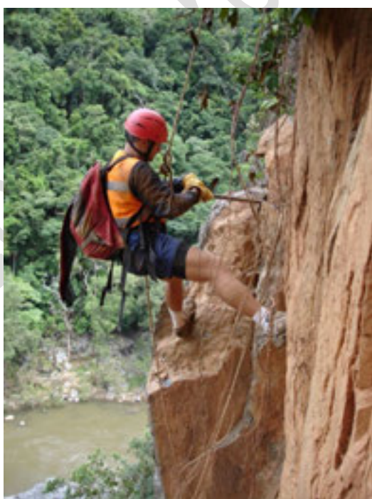
Cairns Regional Council: Dangerous rock removal (scaling) above Macka's Bluff in Lower Barron Gorge
